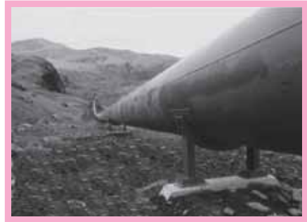
Non-Standard EasiSlide Bearings on Cym Dylli HEP Station, Gwynedd, Wales.
